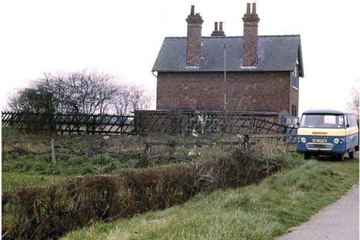
Menthorpe Gate crossing keeper's house in April 1976. The original fence at the back of the down platform can be seen sloping down the platform ramp to the right. Although the fence was still there the platform had long gone by this
