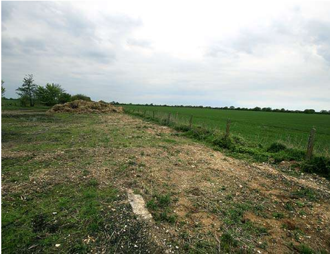
The site of Menthorpe Gate up platform (looking west) in May 2010. The footings of the platform can still be seen.
