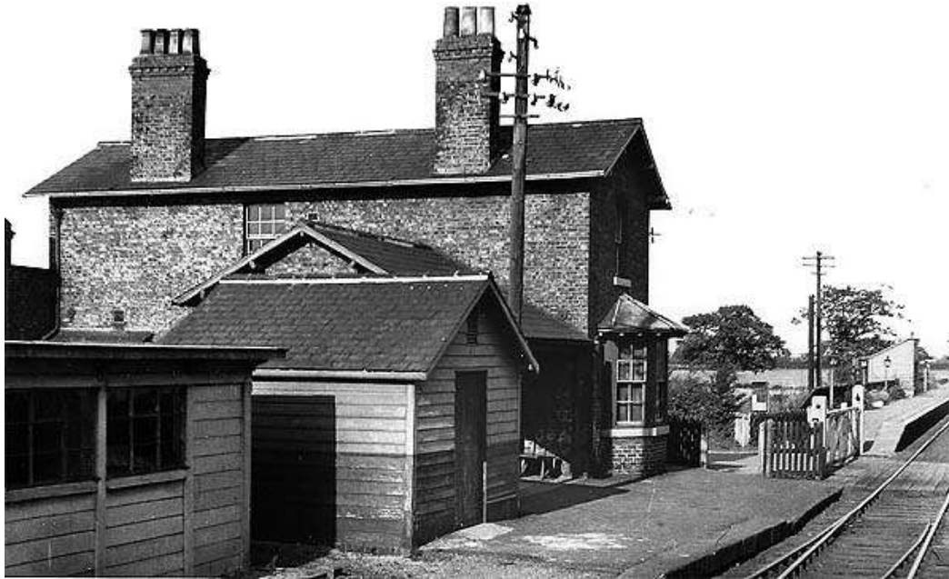
Bubwith station a small low platform in front of the station buildings. This was not for boarding trains; passengers used conventional height platforms which were sited on the far side of the crossing. The down platform is seen here looking east c. early 1950s.
