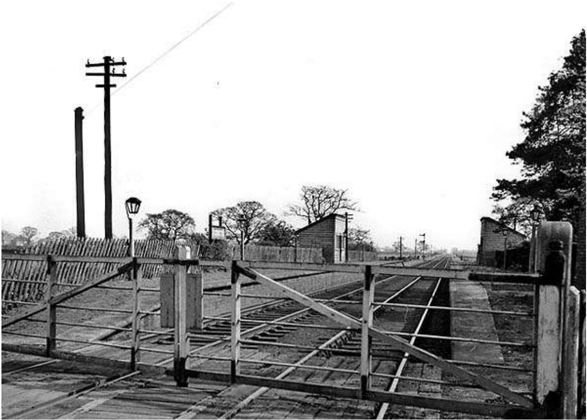
Bubwith station looking east in April 1961.
