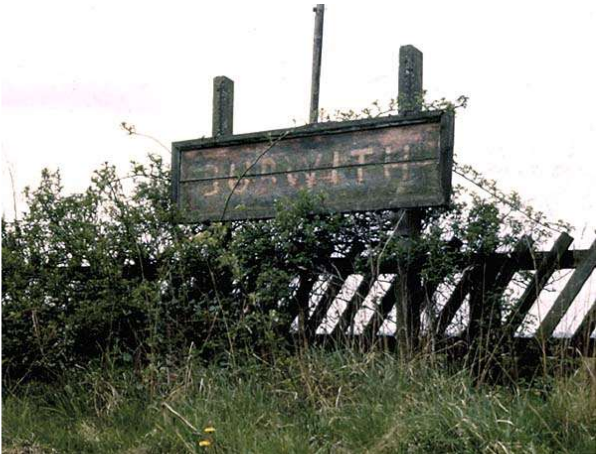
Name board still in place on the up platform in April 1976. Notice how the nameboard is apparently too small for the 'grips' on the stanchions. Unlike that at High Field it isn't the original NER board: it was probably installed by the LNER, but not one of their raised letters type.
